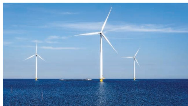
Offshore wind is a proven, reliable, and cost-competitive energy source that is playing a crucial role in the global energy transition.
